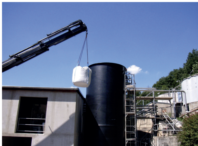
Illustration | Below | BigBag being transported by crane. © Mutag
