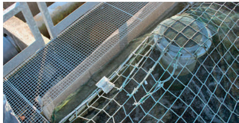
Illustrations | Above | Mesh added on top of an open basin in a fish farm © Surfrider Foundation Europe
